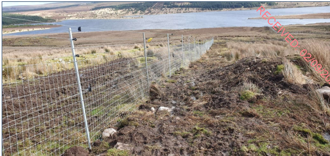
Plate 3-2. Example predator-proof fencing broadly in-line with proposed specifications (for illustrative purposes only) 10 .
